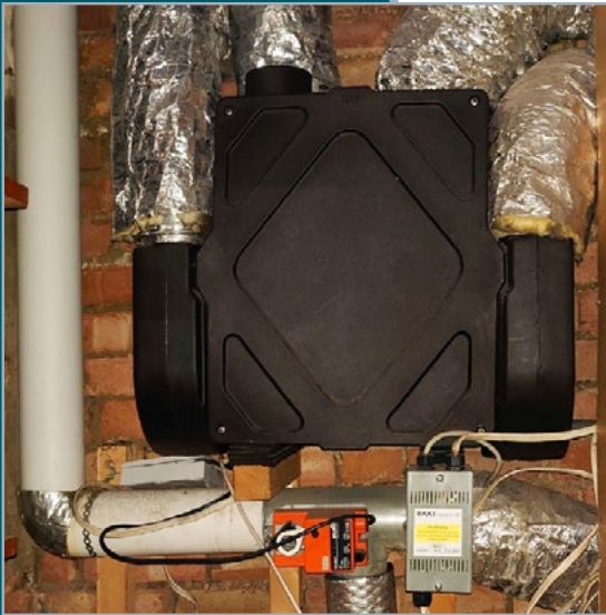
Figures D.5 and 6 Simple MVHR unit with plastic heat exchanger
