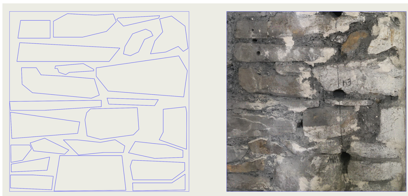
Figure 3. Surface area analysis to determine mortar:stone ratio for the Church Street wall.
